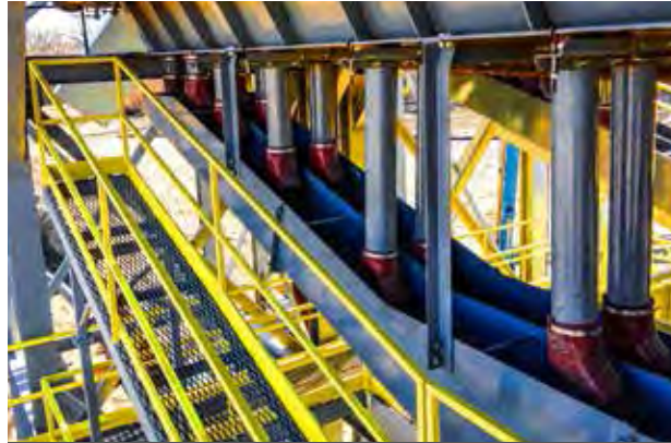
WALKWAY TO ACCESS BLENDING FLUME
