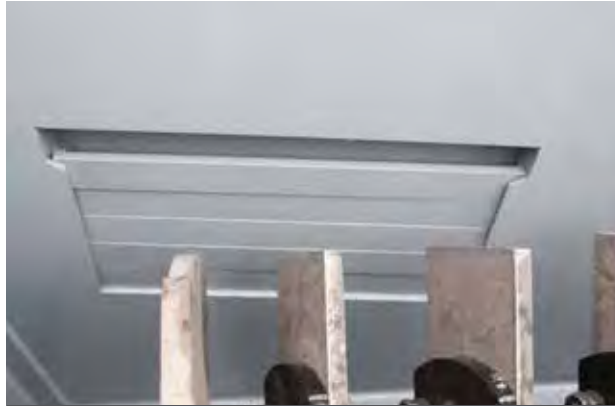
ADJUSTABLE OVERFLOW GATE
