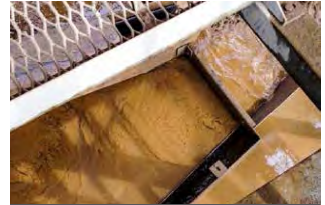
LOAD ZONE BAFFLE SETTLES FINES
