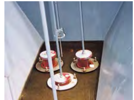
URETHANE DISCHARGE VALVES
