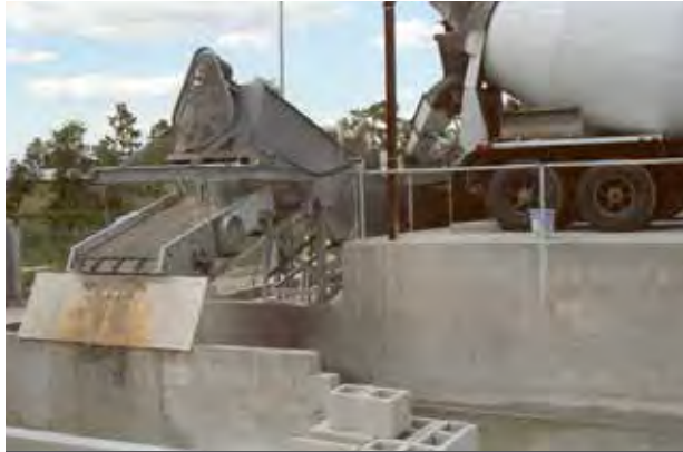
UNLOAD TWO READY-MIX TRUCKS AT ONCE
