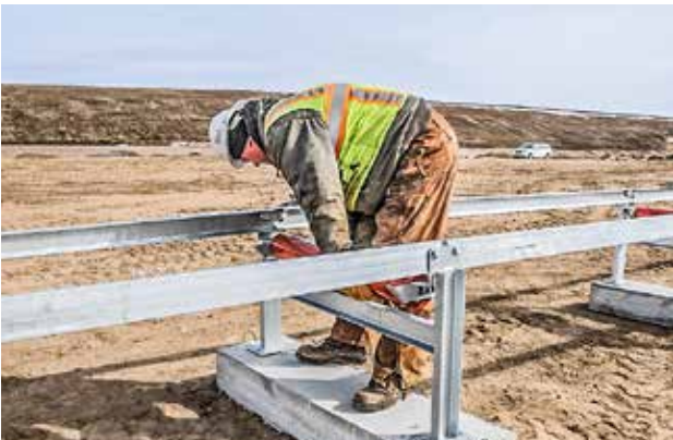
INTEGRATED RETURN IDLER BRACKETS
