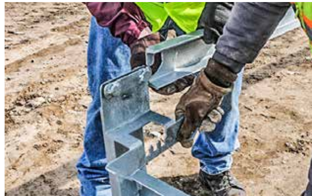
CHANNEL SECTION CONNECTING TO STAND
