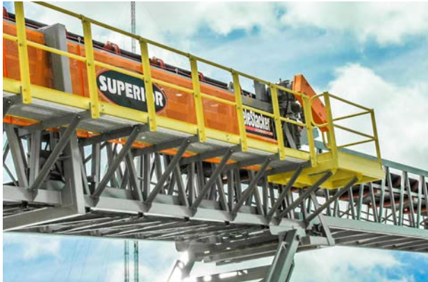
WALKWAY (ON MAIN CONVEYOR)
