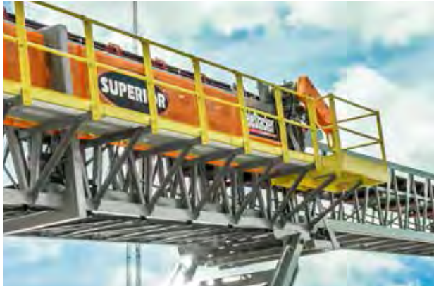
WALKWAY (ON MAIN CONVEYOR)
