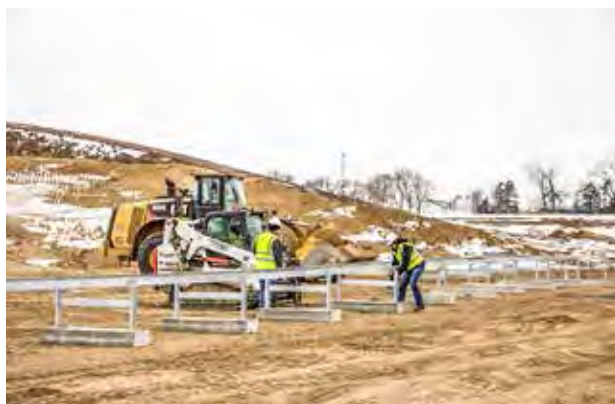
SECTIONS SPAN 10-FEET
