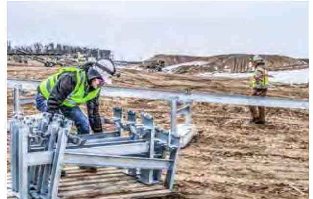
GALVANIZED STANDS AND INTERMEDIATES
