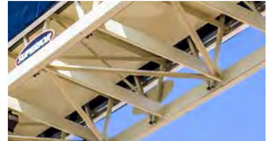
C/ STINGER CROSS BRACING
