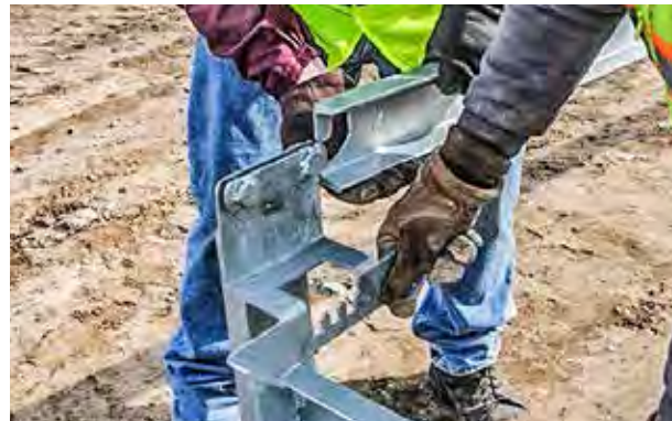
CHANNEL SECTION CONNECTING TO STAND
